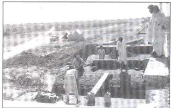
Infrastructure development at Dhabeji
