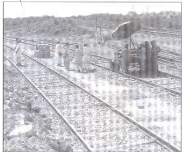
The work begins
